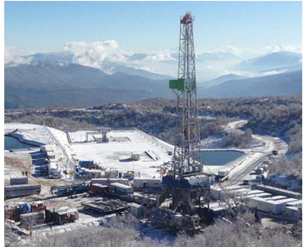
Sarsang drilling rig
