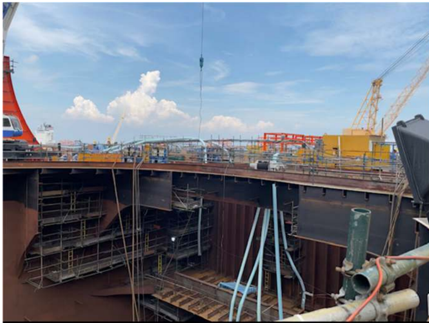
Figure 2-6 View of the large opening inside the tanks for turret mooring to be fitted
