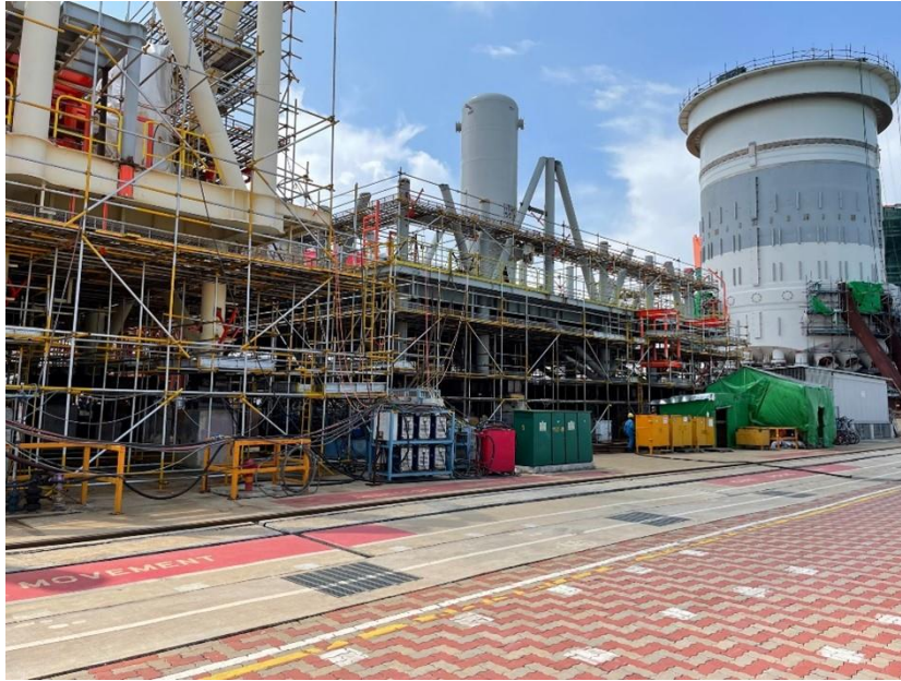
Figure 3-18 Overall view of Module M-20
