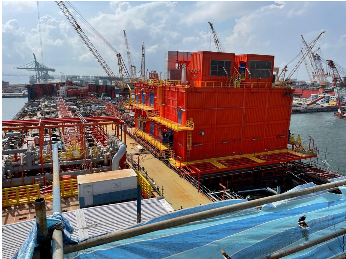
Figure 3-2 Overall View of the deck showing the E-house, metering skid and TMS.
