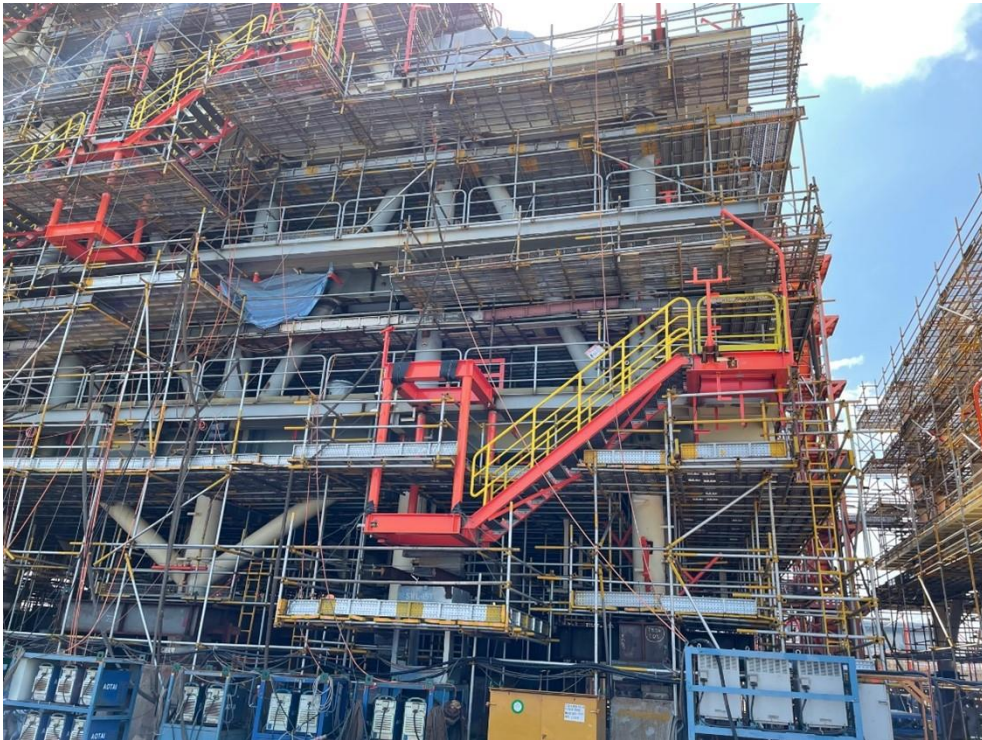
Figure 3-16 Overall view of Module M-30
