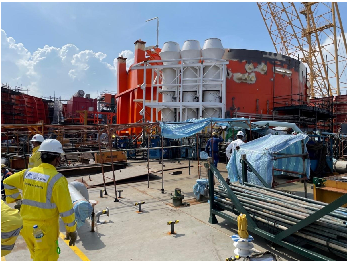
Figure 3-11 View of TMS cylinder
