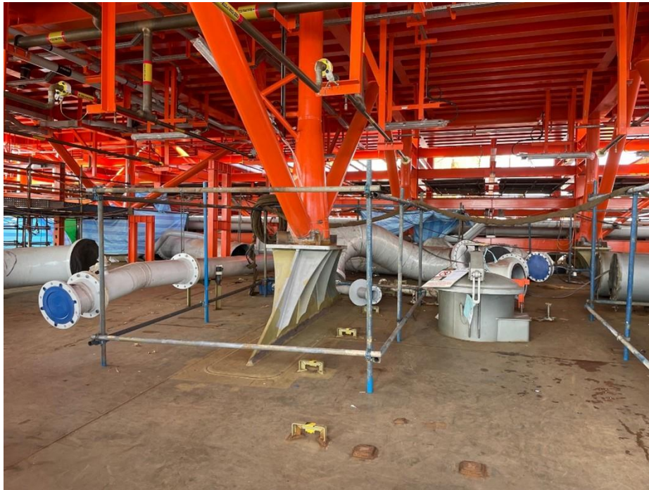
Figure 3-10 Underdeck view of Module M90 – metering skid
