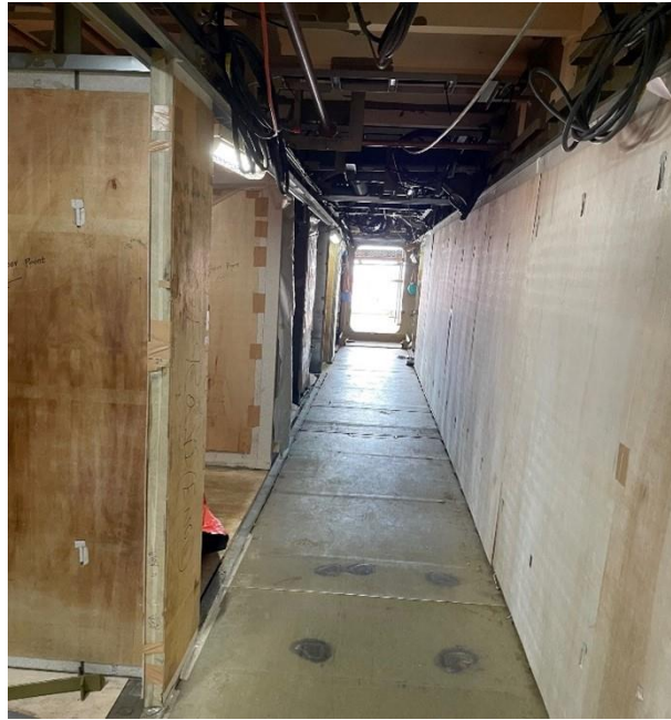
Figure 3-1 View inside the accommodation showing the panelling
