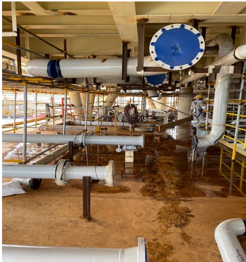
Figure 3-21 Another inside view of Module M30
