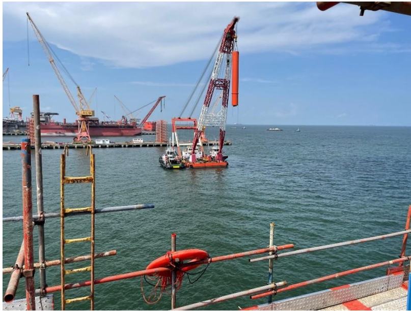
Figure 3-14 Crane pedestal ready for installation on deck
