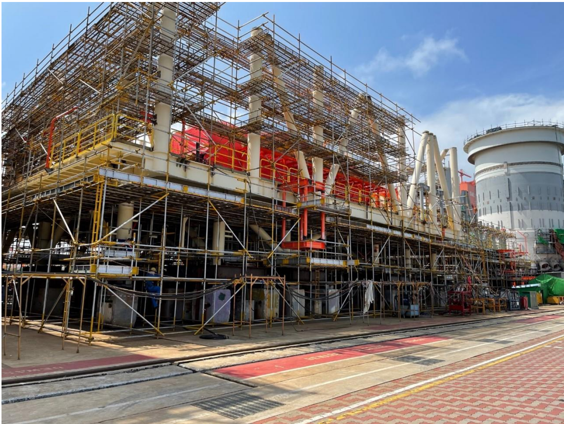
Figure 3-17 Overall view of Module M31
