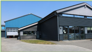
North Tec Location: Bredtstedt, Germany
